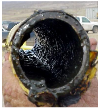
Pipe after SpiroFlo
