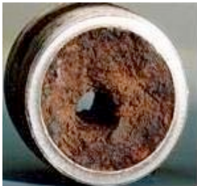
Typical paraffin clogged pipe
